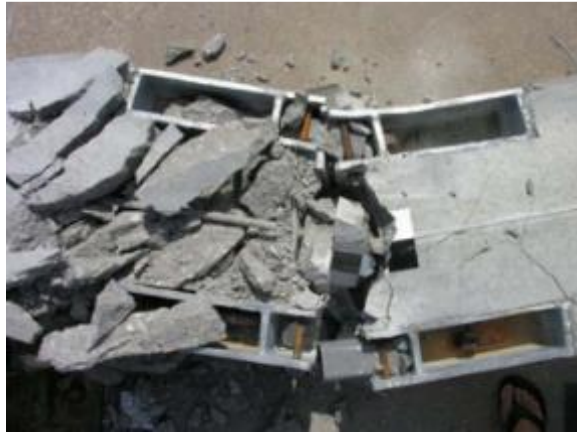
Figure 2.19 Side bolt and shear tube connection failure ( MWRSF, 2012 )
