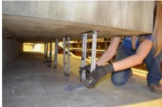
Figure 4.19 Insertion of U-bars
