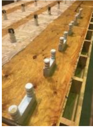
Figure 4.8 Deck block outs to facilitate U-bar installation
