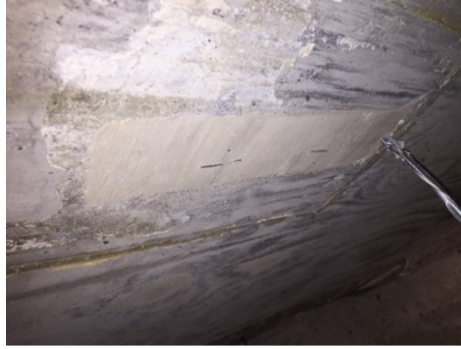
Figure 4.23 Finished U-bar grout pocket
