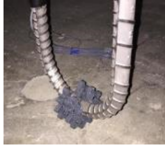
Figure 4.18 Rebar Chairs for #7 Bars
