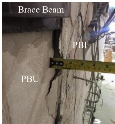
Figure 5.29 Difference in barrier movement at barrier to barrier connection at the maximum load during Test 4
