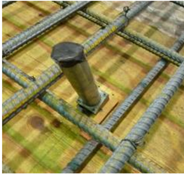
Figure 4.10 Installed PBI connection sleeve with deck reinforcement
