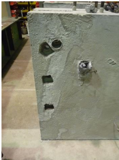
Figure 4.16 Pockets used to install transverse barrier to barrier connection
