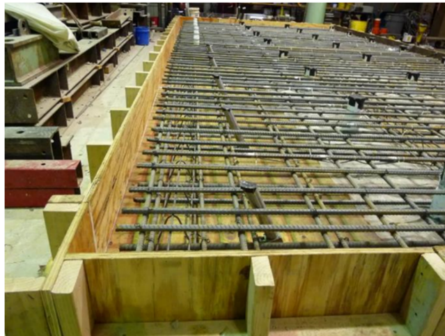
Figure 4.9 Bridge deck reinforcement
