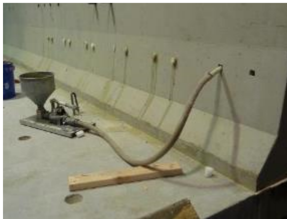
Figure 4.22 Grouting of U-bar pockets
