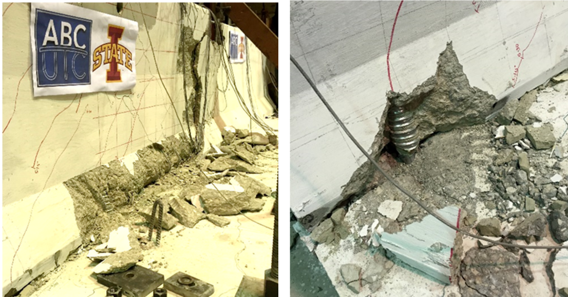
Figure 5.36 Concrete spalling on front of PBI at deck interface and barrier to deck connection
