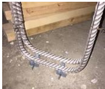
Figure 4.17 Rebar Chairs for #5 Bars
