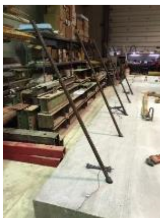
Figure 4.14 Inclined reinforcing bars connected to bridge deck before placement of precast barrier
