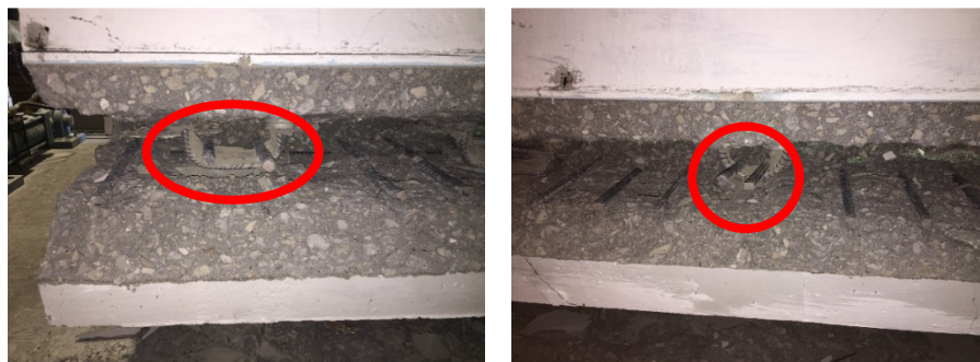
Figure 5.41 Top matt of the bridge deck reinforcement after the Test 6 pull test
