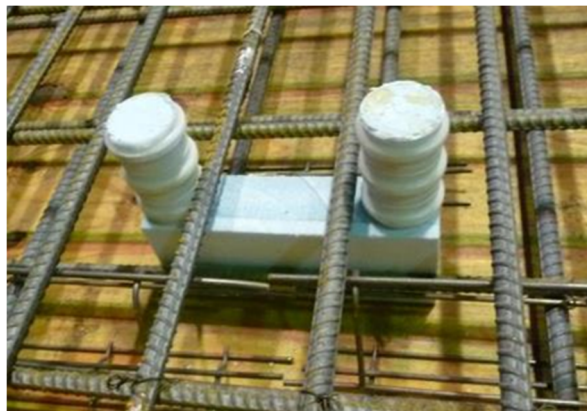
Figure 4.11 U-bar access blocks out with terminated bottom deck steel and top deck steel positioned to be within a u-bar connection
