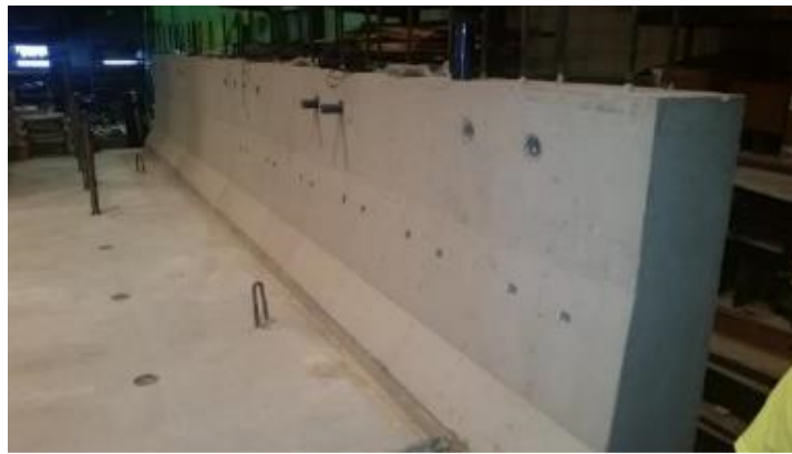
Figure 4.24 Completed barrier installation
