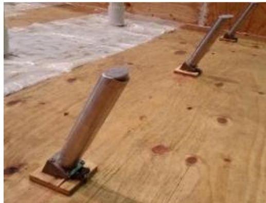
Figure 4.7 Connected inclined receiving end piece to the deck formwork
